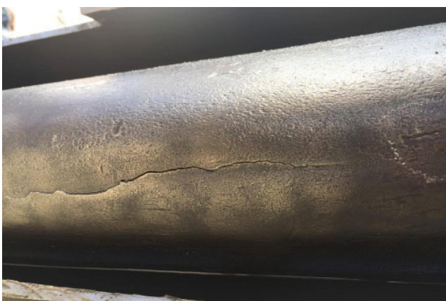
Figure 6 Photo of a fragment of the inner pipe in the defect zone, the location of which was determined by the AE method Slika 6. Fotografija dijela unutrašnje cijevi u oštećenoj zoni, čija lokacija je otkrivena AE metodom
