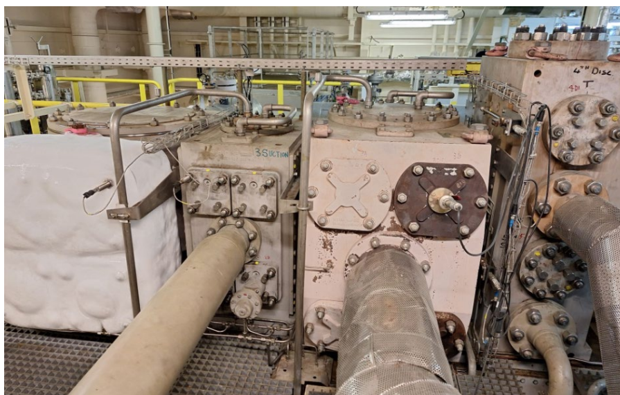
Figure 1 Burckhardt Compressor, model 5LP250-5B-1
