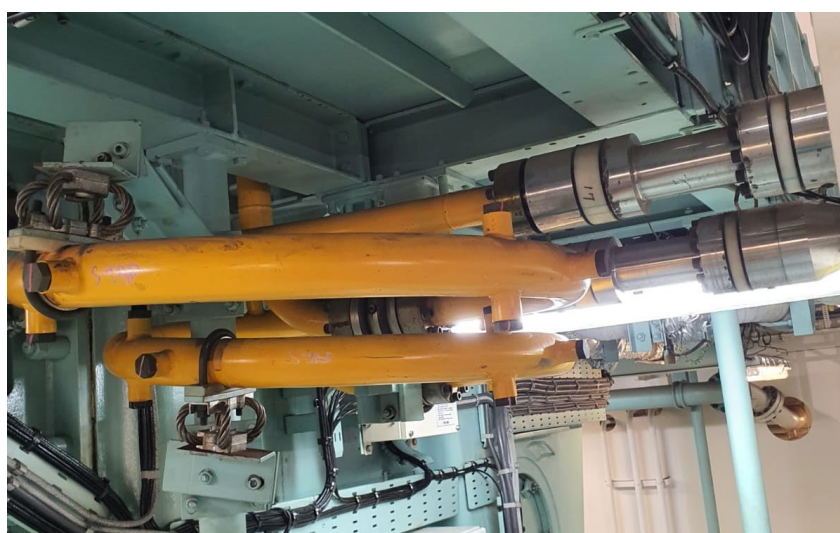
Figure 4 Helix pipe – compensator
